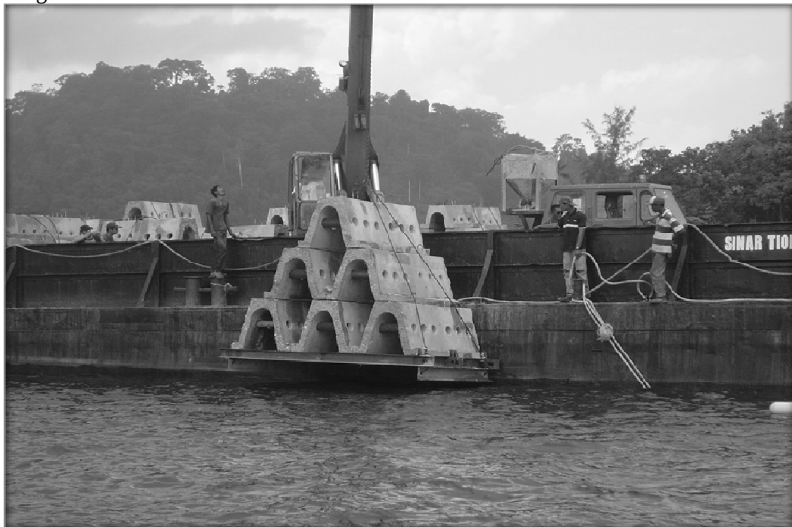
Figure 1: WABCORE artificial reef being deployed for the first time in Panuba Bay, Tioman Island
