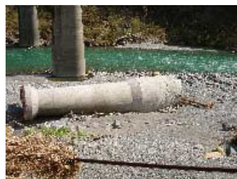
Fig. 9 Collapsed RB 3 of the Asuwa River Fig. 10 Collapsed RB 2 of the Gokase River
