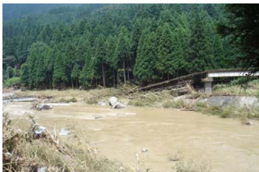
Fig. 9 Collapsed RB 3 of the Asuwa River Fig. 10 Collapsed RB 2 of the Gokase River
