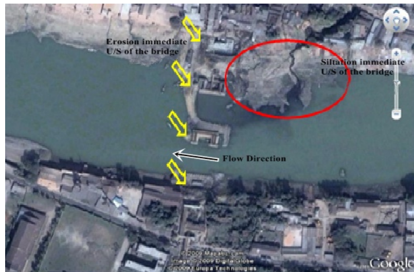
Figure 5: View of the bridge site showing erosion and siltation
