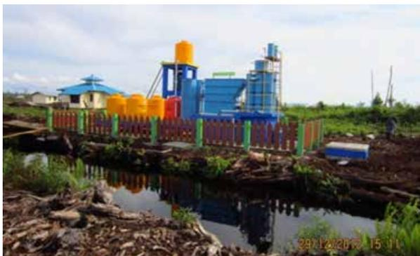
Figure 7.1.9. IPAG 60 : from peatwater to clean water. Photo ©APCE
